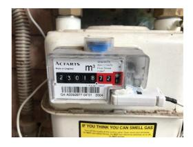
Measure the Energy consumption of Main Incoming Utility supplies. Identify actual consumption from Gas, Water and Electricity usage by remotely reading compatible meters.
